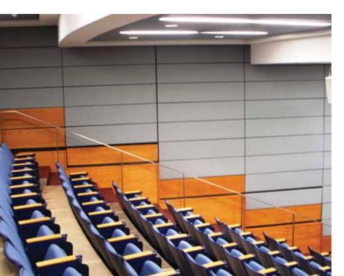
**INTEGRATED DESIGN CONCEPT** The project team used the retracted Skyfold walls as part of the ceiling detail.
